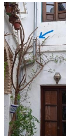
PHOTO 4. AIR QUALITY. PATIO 22 FIRST FLOOR
